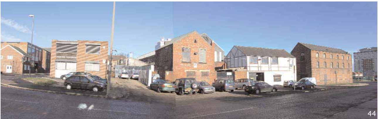
Poor quality edge to southern boundary of Tavistock
