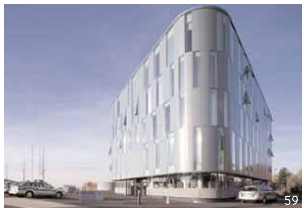
An appropriate response will be required in key gateway sites
