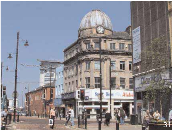
Mackie's Corner, Fawcett Street
