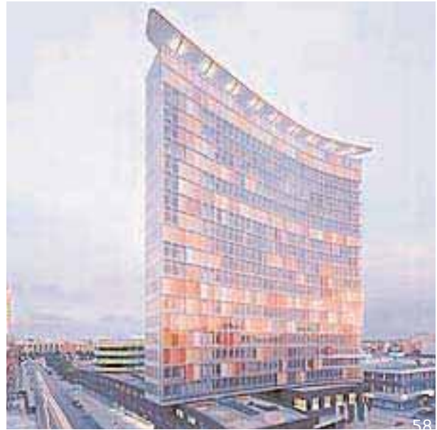
Taller buildings can be used to reinforce key gateways
