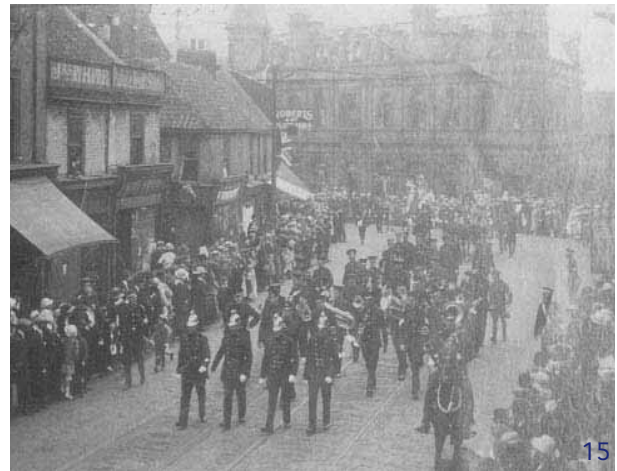
High Street West
