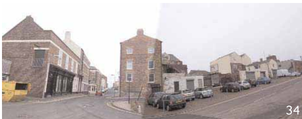
Low quality environment within the North East Sector (view south down Sunderland Street)
