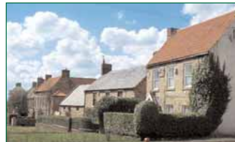
Natural slate and clay pantiles are distinctive roofing materials of local architecture. The photograph illustrates how varied roof heights add to the character of the area.
