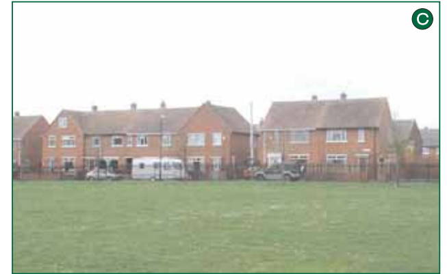
Western boundary of site.
