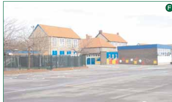
View of existing school buildings.
