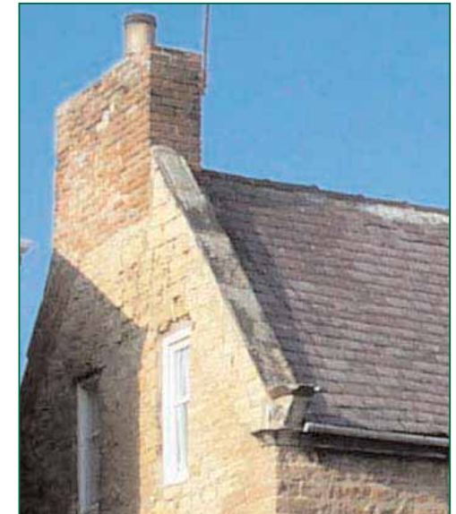
An example of a traditional style dwelling, found throughout the coalfield area, with slate roof, sash windows and simple door surround.
