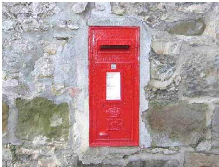
Left: although the post box is a charming and attractive feature of the wall on Warden Law Lane, the way it has been inserted into the wall has resulted in an unsightly area of poorly finished cement mortar, which may also be causing some damage to the surrounding stonework. Note the greenish discolouration on the stone to the bottom left of the post box; this is probably evidence of dampness due to water entering the stone, rather than the adjacent mortar.
