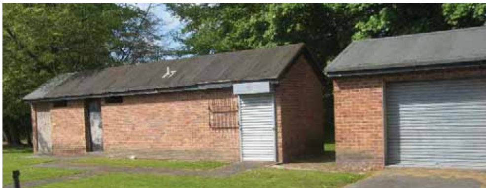
Above: the now apparently disused toilet block to the north-west of the park is of very poor appearance and detracts from the park's special interest.
