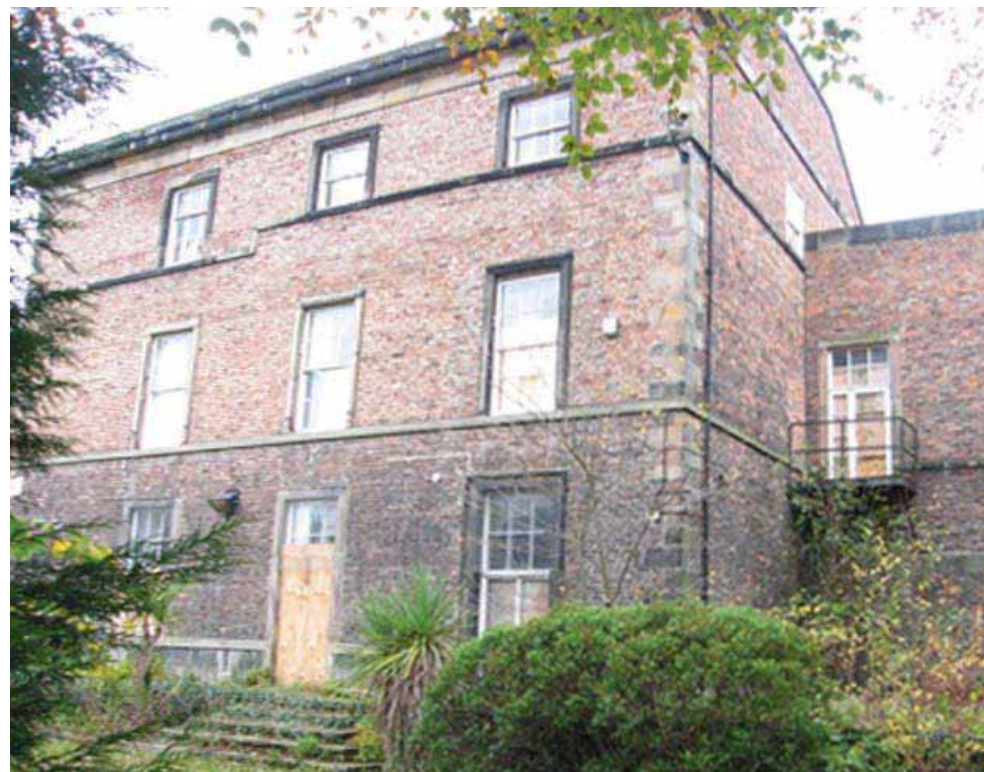
Doxford House October 2009. The building is vacant and deteriorating with doors boarded-up and window panes cracked or missing.
