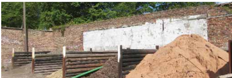
Above: the western half of the walled garden is currently used as a maintenance depot. The white section of the wall indicates the location of a structure, probably a glass house.
