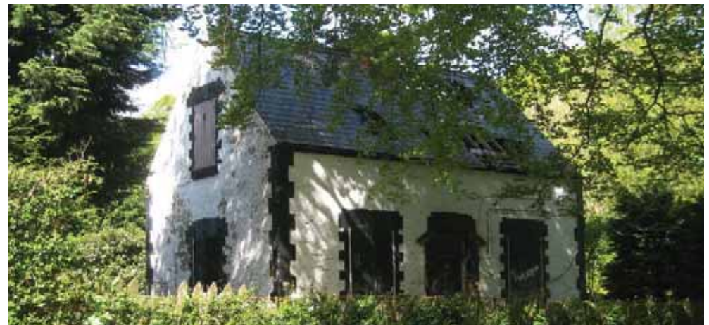
'The Gardens', sadly derelict, but of considerable historic interest.
