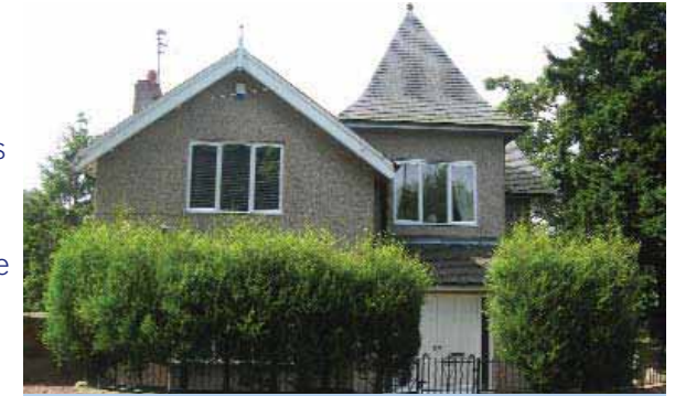
The Lodge, Silksworth Hall Drive
