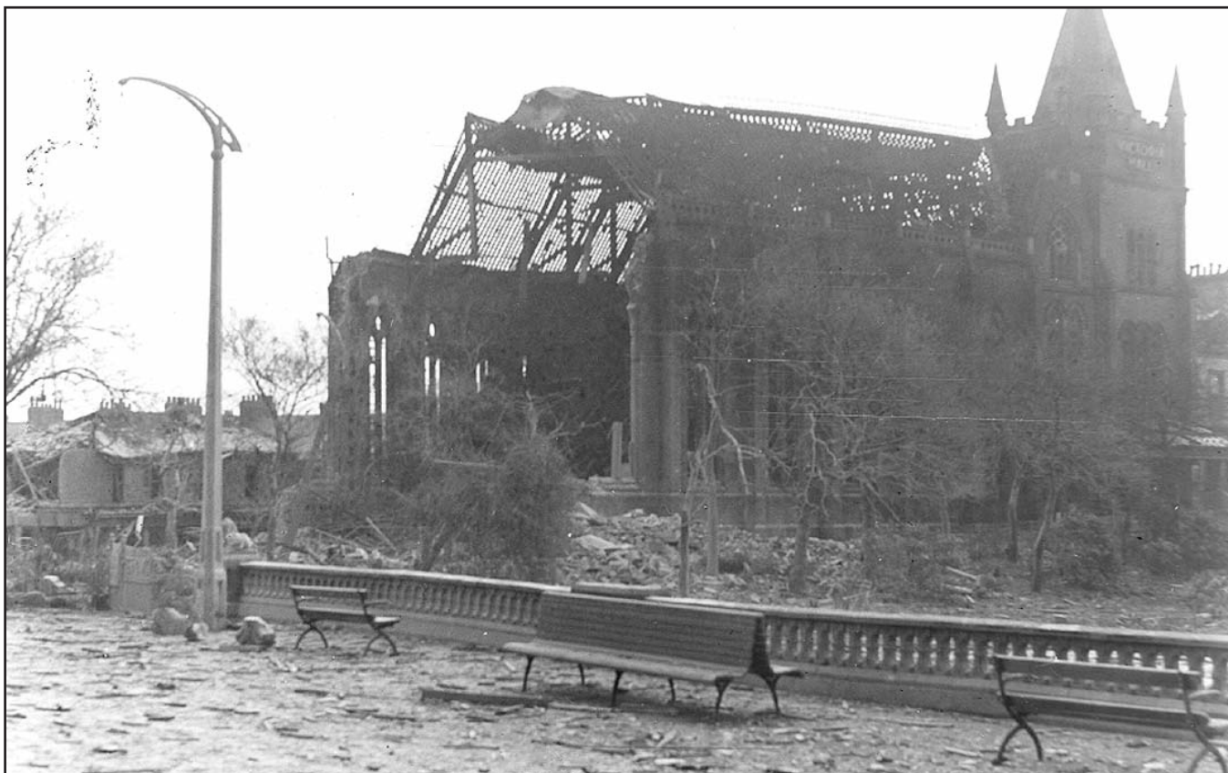
The bomb damaged Victoria Hall in 1941
