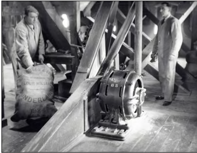
EB & TC AT INTAKE PLANT
