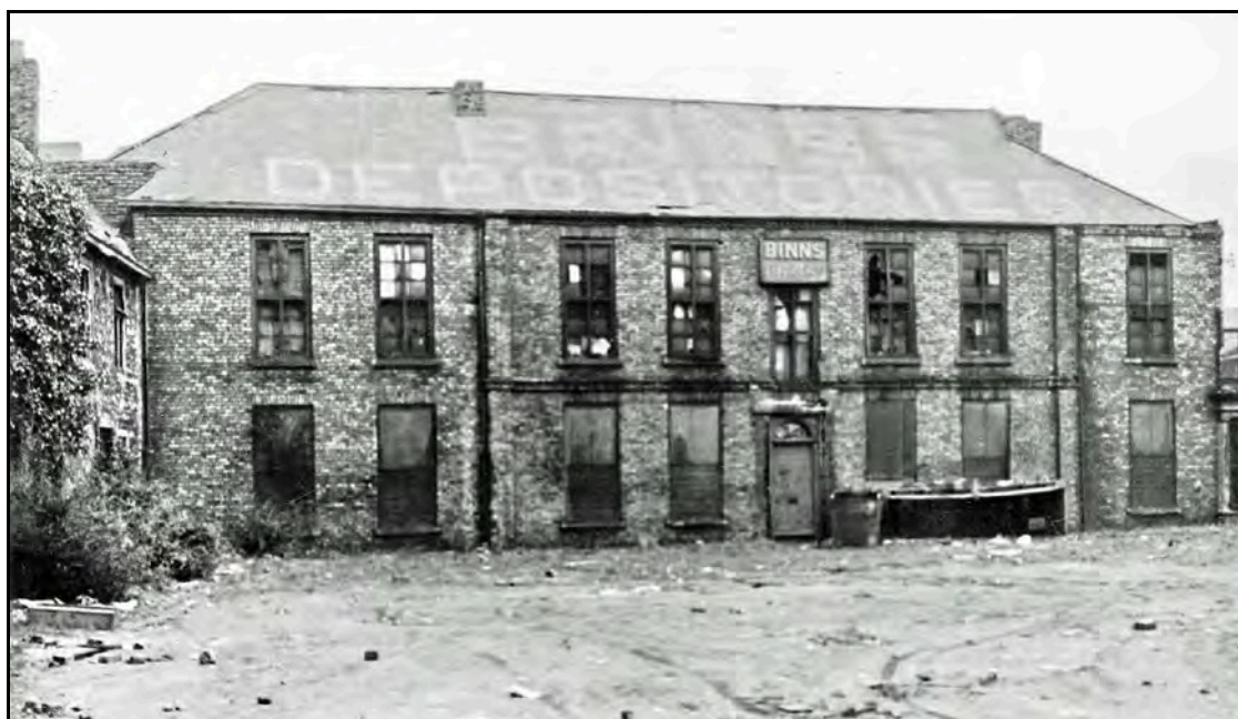
The west face of Fenwick Lodge viewed from the Green
