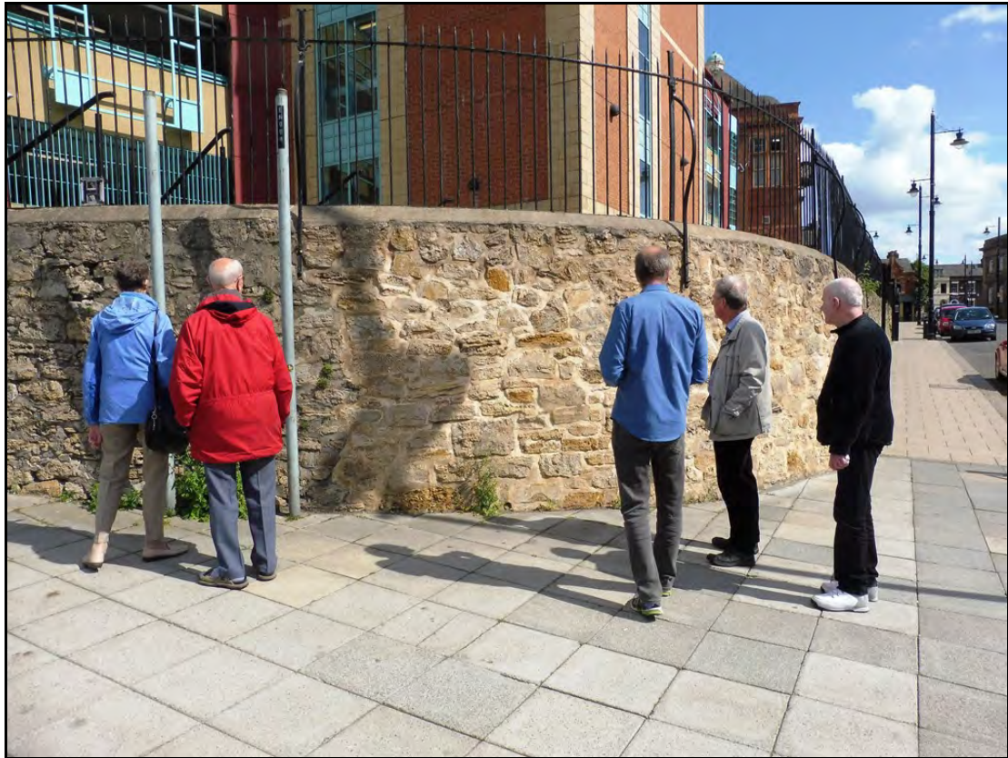
The retaining wall being examined by the Atlas Study Group
