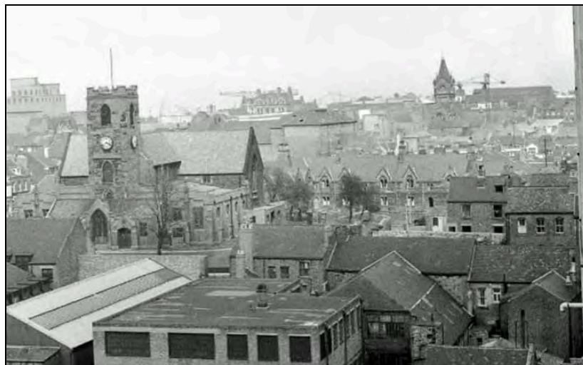
Oblique aerial photograph of Southgate from the west, date unknown
