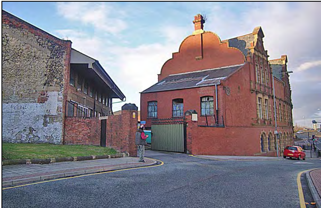
A 2014 view of the Sunderland Corporation Gas Company offices and showroom with the associated retort building (since demolished) to the left.
