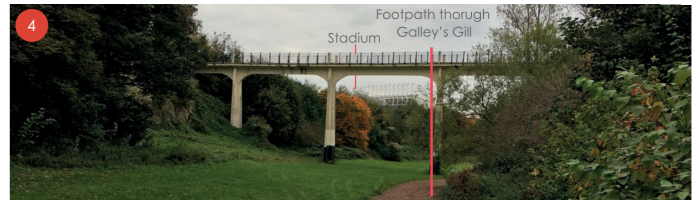
Pic.4 View from Riverside Park looking north towards Stadium of Light
