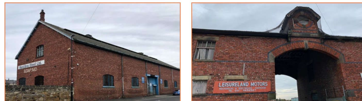
Figure 29 - Image of the Engine Shed, and the Grade 2 listed former stables.
