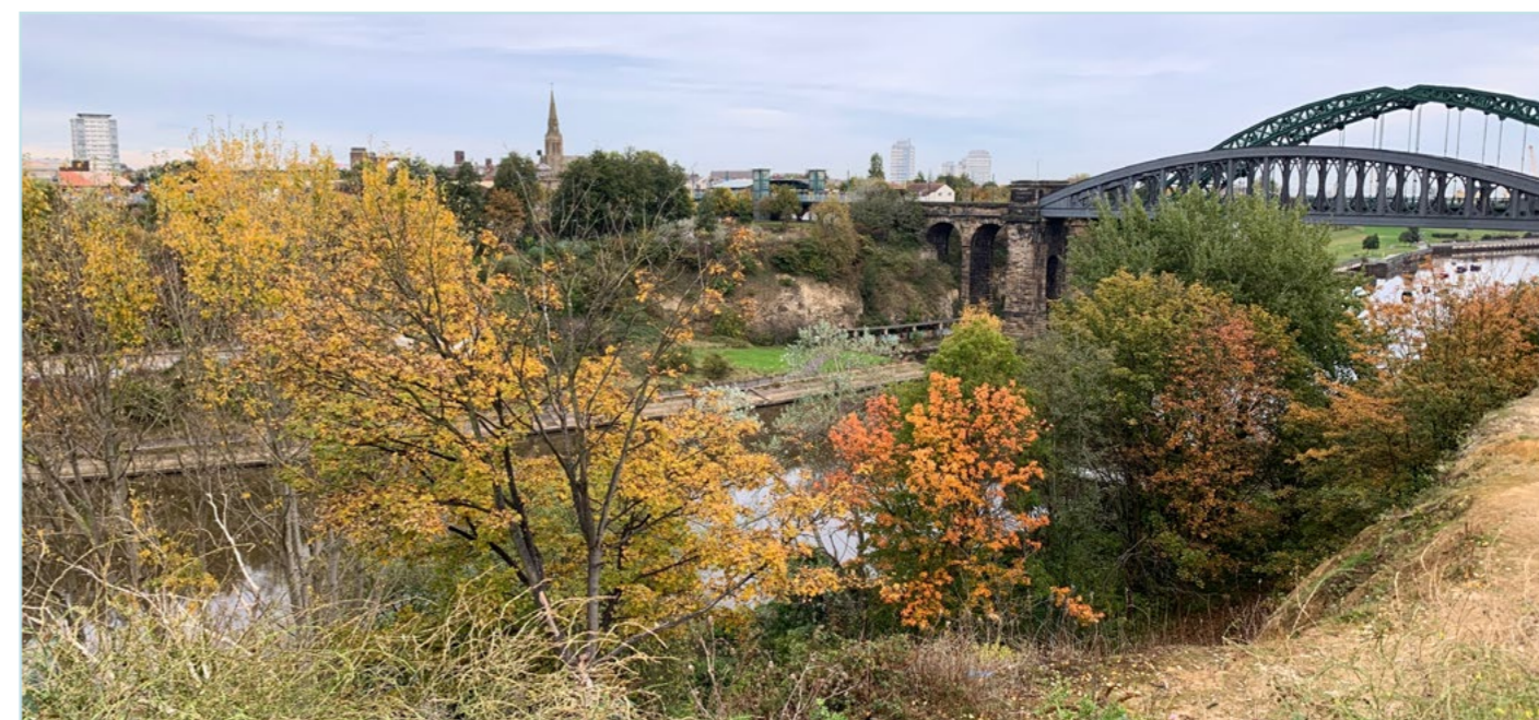
Figure 37 - View towards Monkwearmouth Railway Bridge
