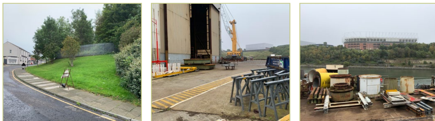
Figure 25 - Images of existing buildings
