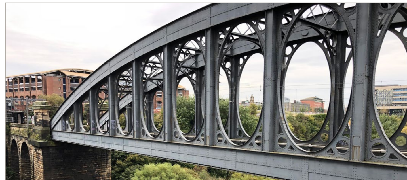
Figure 31 - View from Bonnersfield looking through the Monkwearmouth Railway Bridge heritage asset
