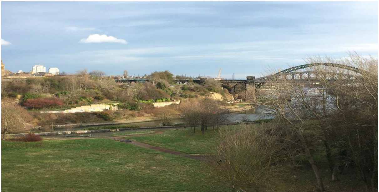
Figure 62 V61: North and East across River Wear valley towards Stadium of Light from Festival Park viaduct
