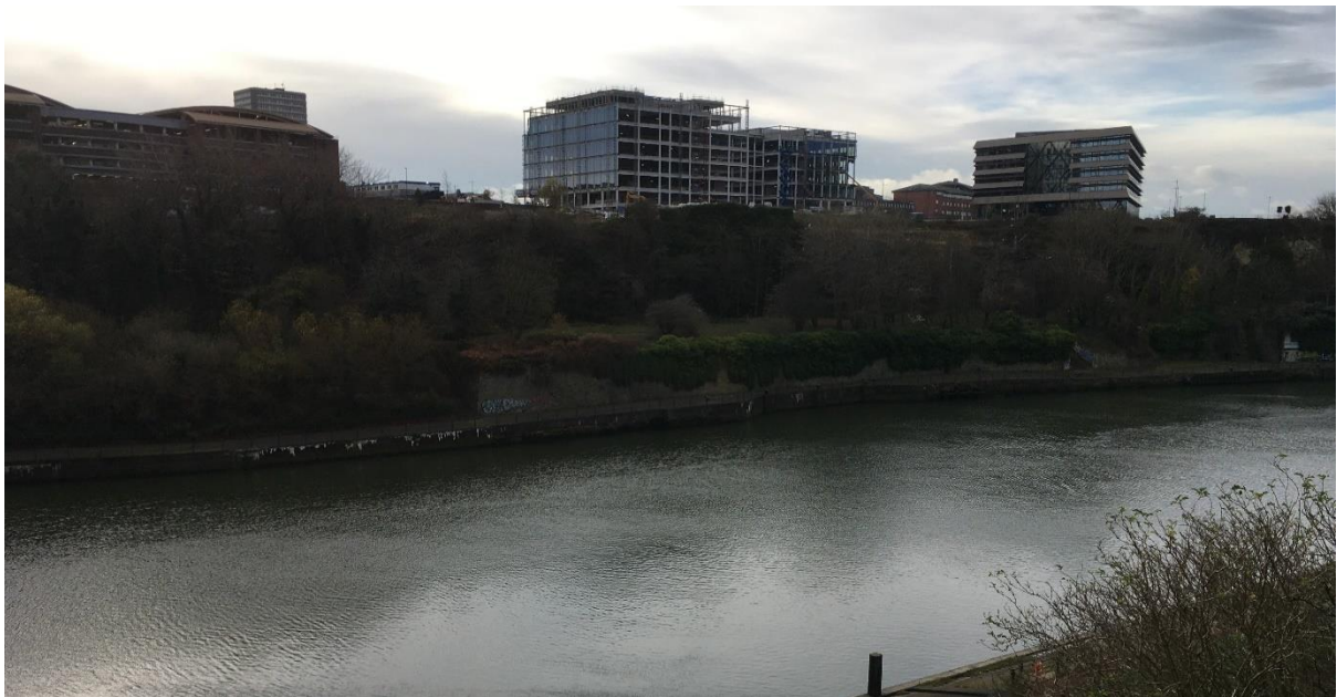
Figure 66 V65 West along the River Wear valley from Wearmouth Bridge
