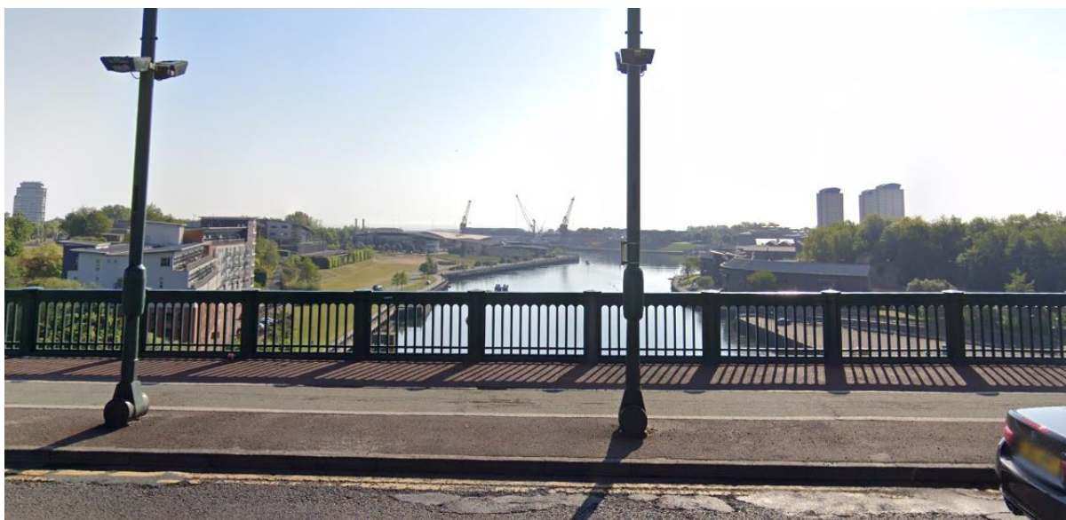
Figure 67 V66: East along the River Wear estuary from Wearmouth Bridge
