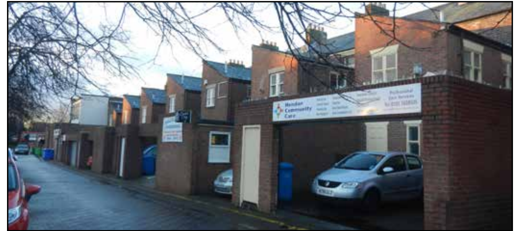
Coordinated extensions to the rear of Mary Street reinforcing the rhythm of the terrace
