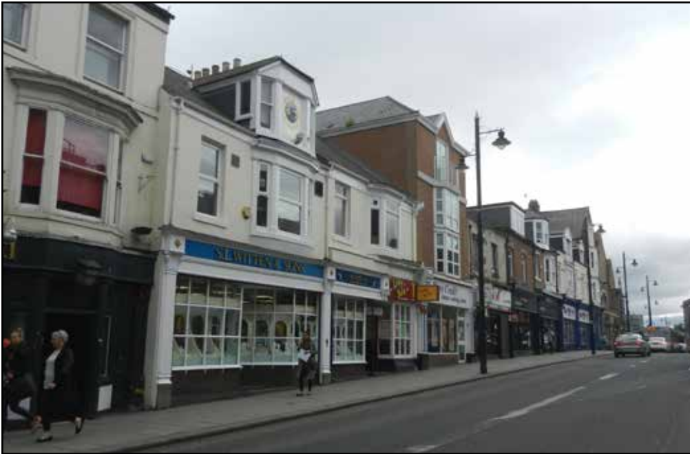
A mix of window styles can be seen on Vine Place
