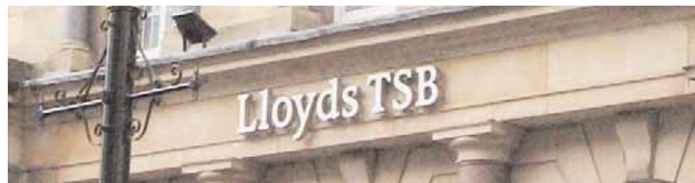
Above: freestanding individual lettering on a Listed sandstone building minimises the impact of the commercial signage on this historic property. Although the signage is not in the Bank's usual style and is devoid of corporate colours and logos, it is nonetheless distinctive and easily recognisable, demonstrating that a sensitive conservation-led approach to signage does not jeopardise the advertising potential of a business.
