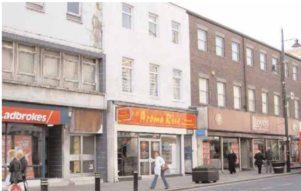
Poor quality modern shop frontages on Fawcett Street. The property on the left can also be seen to be suffering from a lack of maintenance above ground floor level.
