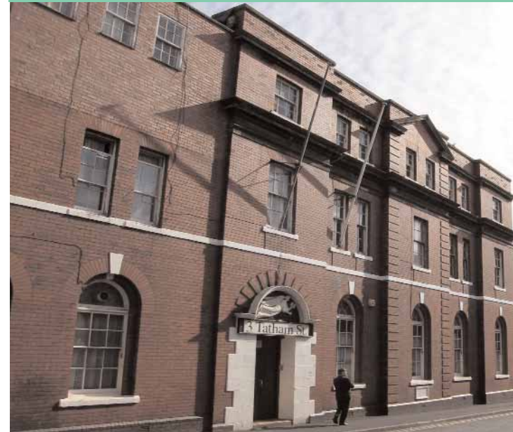
3, Tatham Street - former girl's reformatory and Seamen's Mission
