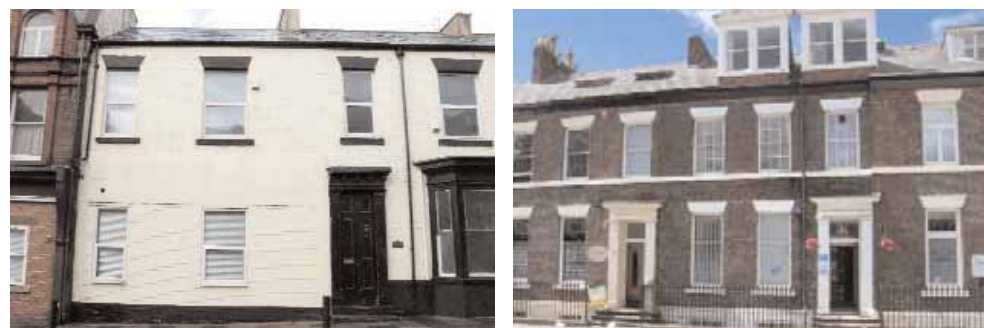
Above: uPVC windows in an historic property (left) fail to accurately reflect the elegant proportions of traditional timber sliding sash windows (right).
