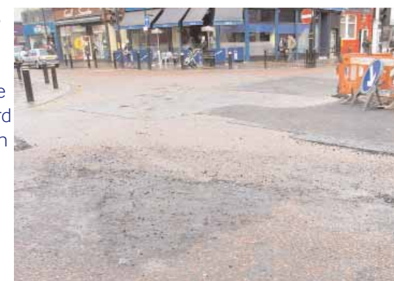
Above: poor street surface on Fawcett Street and buildings presenting a negative appearance on the upper floors.
