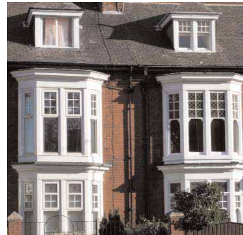
The visual impact of uPVC windows in an otherwise uniform terrace
