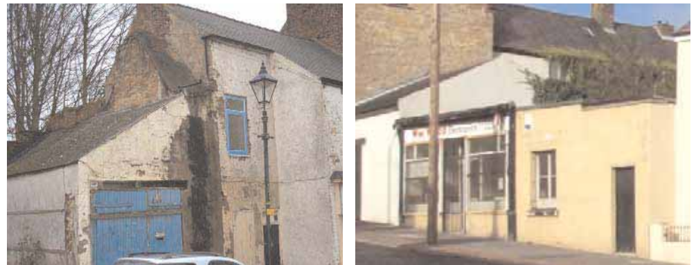
Left: this building has been deteriorating for some time and is in need of some repair work; right: a small cluster of relatively modern flat roofed buildings create a contrast against the historic properties of Nesham Place; these properties could benefit from improvement works
