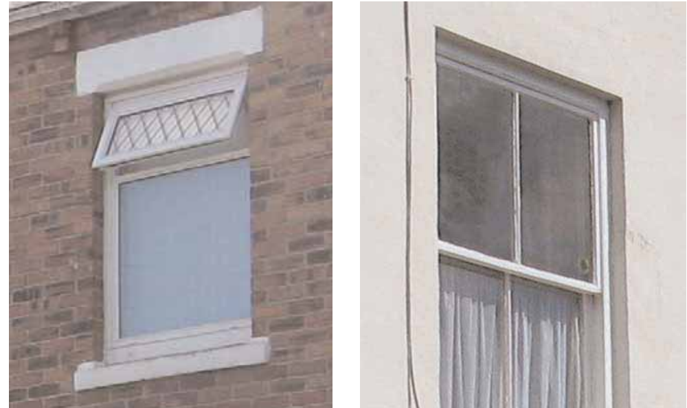
The replacement uPVC window to the left fails to match the slender proportions and historic detailing of the traditional sliding-sash in the property to the right. Such alterations are inappropriate for historic buildings and contrary to the aims of the Article 4(2) Direction.
