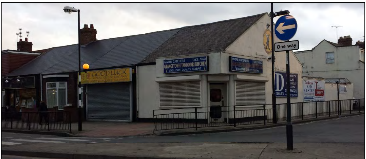
Photo 5: Shows the set of two adjoining takeaway units within Grangetown Local Centre
