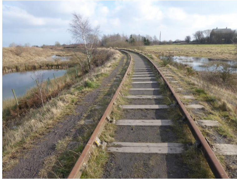
Railway line adjacent to the site with Ponds P1 and P2
