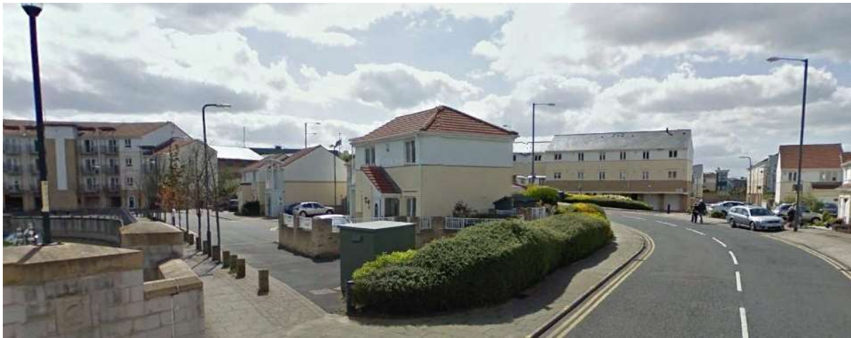
Figure 28. Captain's Wharf, South Tyneside
