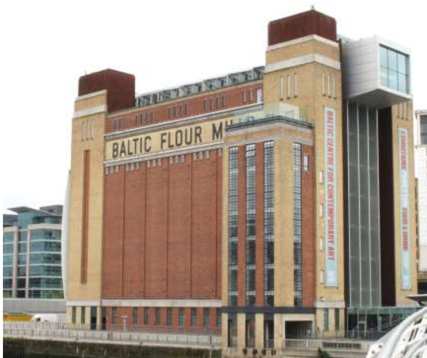
Figure 54. Baltic Flour Mill, Gateshead.
