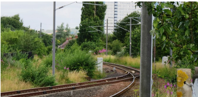
Bensham: Electric power lines over a freight-only line track curving from the Team Valley towards Metrocentre
