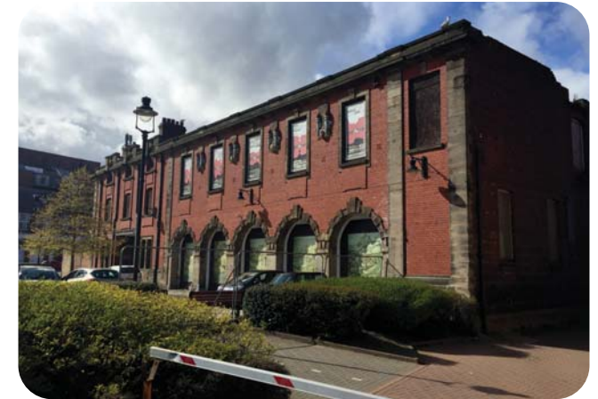
Figure 49: Photograph – Former Fire Station
