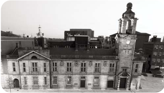
Figure 17: Photograph – Magistrates Courts, Grade II, Listed Building
