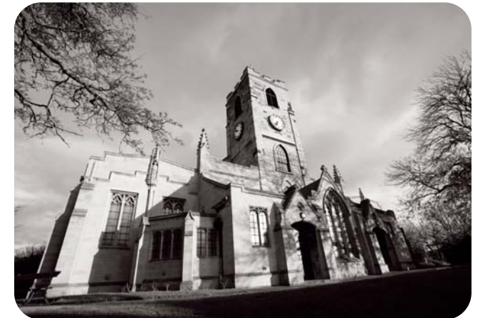
Figure 13: Photograph -Sunderland Minster, Grade II* Listed Building
