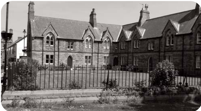
Figure 18: Photograph – Mowbray Almshouses, Grade II, Listed Building
