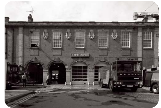
Figure 20: Photograph – Fire Station on Dun Cow Street
