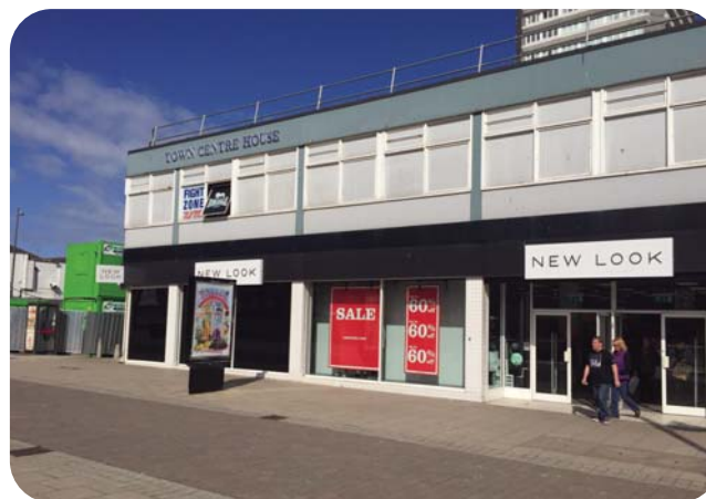
Figure 59: Photograph – Town Centre House
