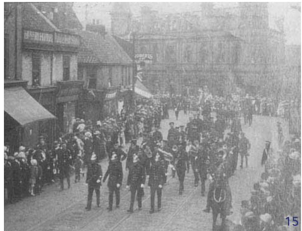
High Street West
