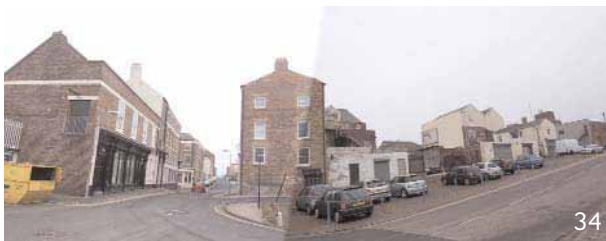
Low quality environment within the North East Sector (view south down Sunderland Street)
