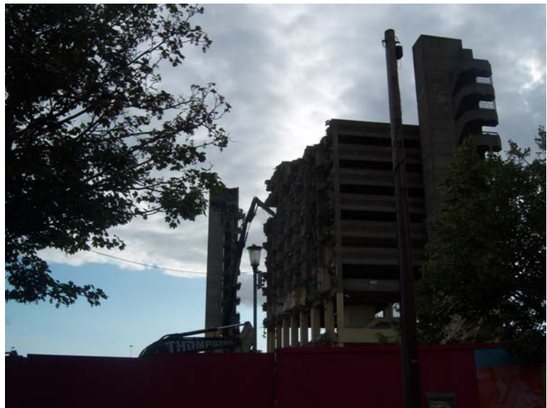
Gateshead car park undergoing demolition
