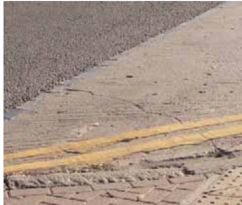
Poor mix of surface materials creates an untidy image.
