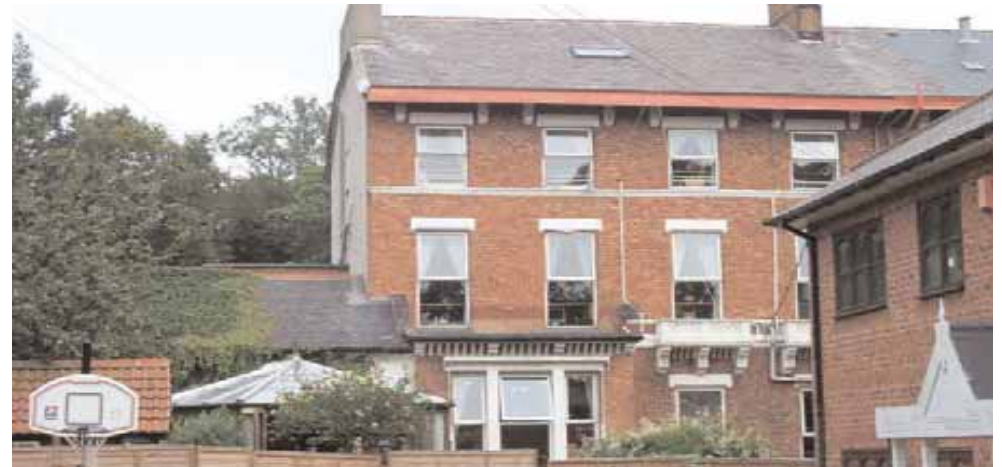
Ashwood House (right) modern infill development to the rear of 4 The Cedars - new properties in such close proximity to historic buildings can compromise the character and setting of a building.
