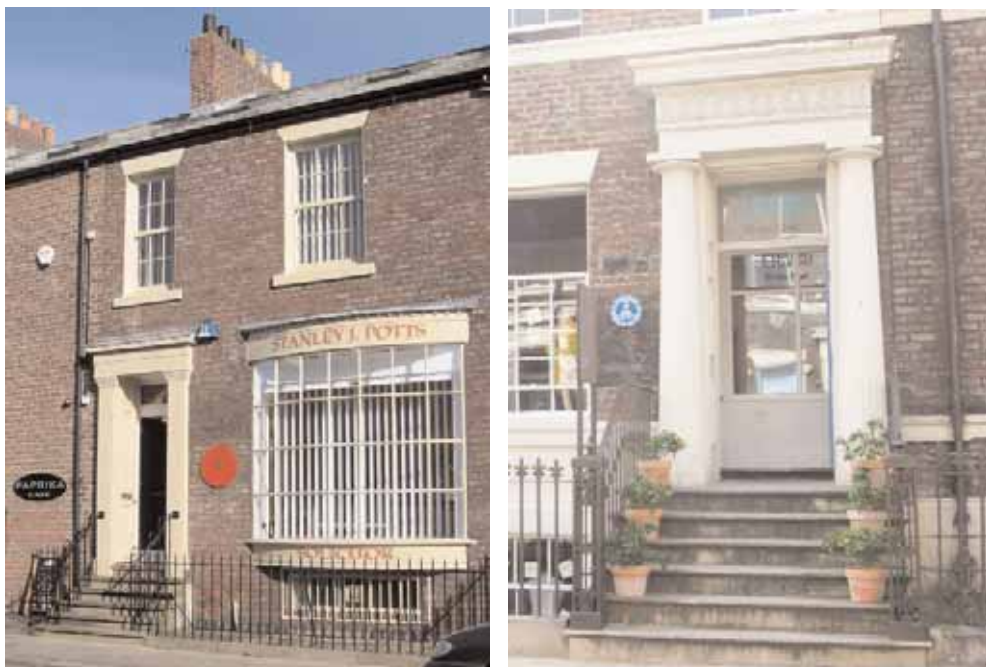
Above left: despite a large shop window, inserted many years ago, this property on Frederick Street has largely retained its domestic appearance: such interventions will not, however, be allowed in future. Above right: this shop on John Street retains all of its domestic characteristics, with subtle signage.
