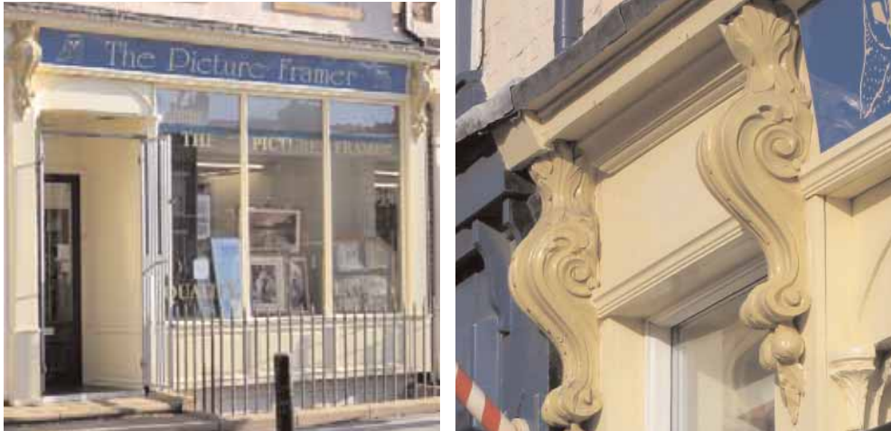
Above: a traditional shop front on Norfolk Street, complete with decorative consoles
