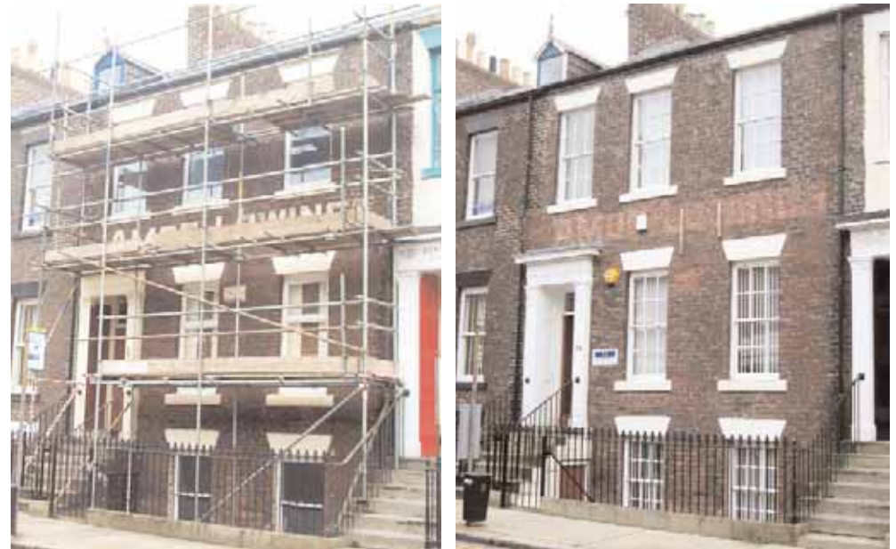
This Listed Building in Frederick Street was vacant and in poor condition, having suffered from alterations that had despoiled its special architectural and historic interest. Funding from the SCPGS secured the full restoration of its frontage, including reinstatement of Georgian sash windows and front door, and the fit-out of its interior to modern office standards. The works enabled the property to be brought back into use as an accountant's office, facilitating the establishment of a new business and the creation of jobs in Sunnyside.
