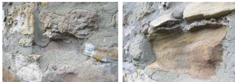
Above: the effects of using too “strong” a mortar - the stone face has eroded behind the level of the surrounding mortar joints, which are left standing proud of the stone
