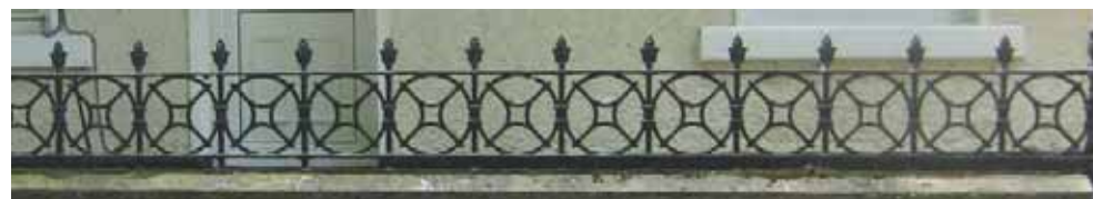
Above: cast iron railings to the Lodge, Warden Law Lane
