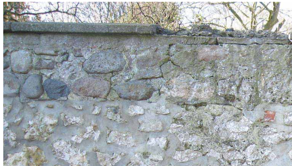
This section of wall on Warden Law Lane has had the original coping replaced, part of which is missing, and features some inappropriate cement pointing
