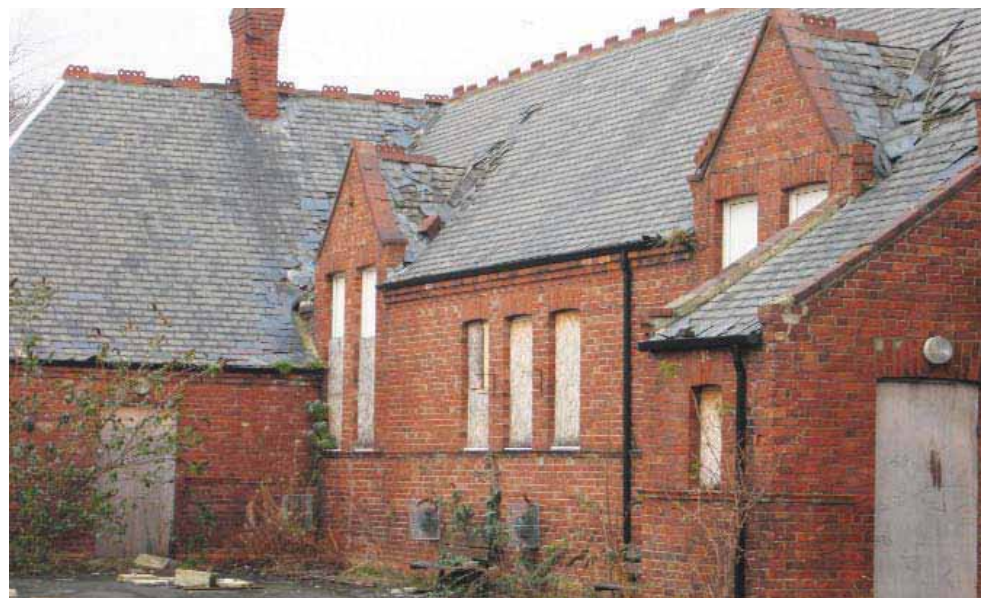
The vacant former village school showing the symptoms of decay and the effects of theft damage, prior to recent repair works being undertaken.
