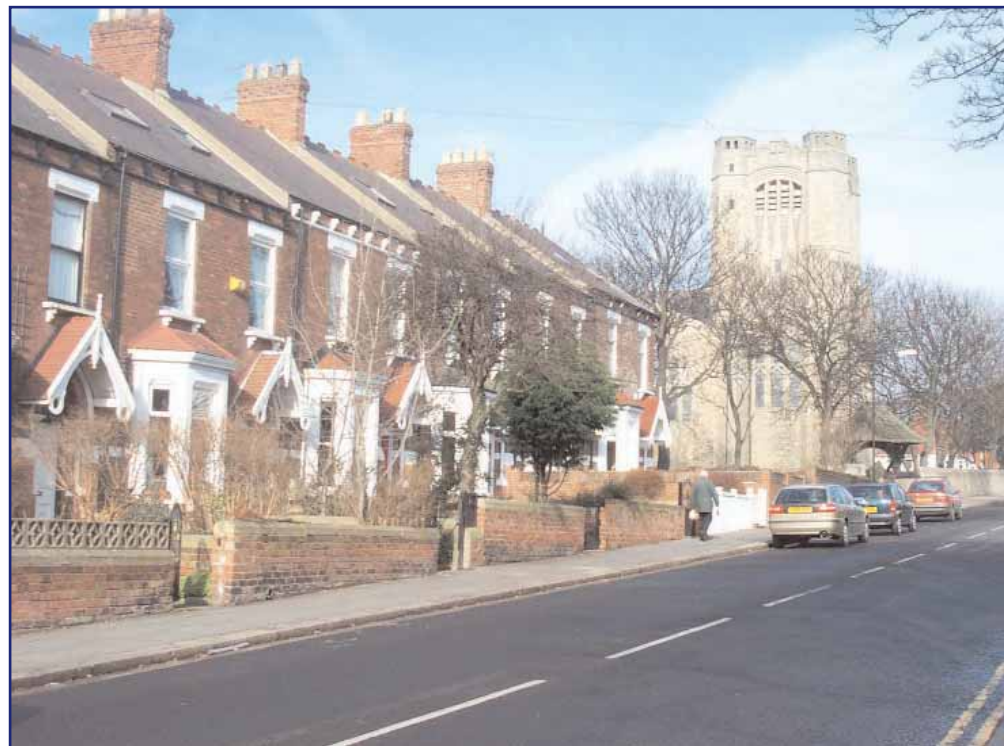
The use of local limestone sets St Andrew's Church apart from adjacent buildings and provides interesting contrast in the street scene.
