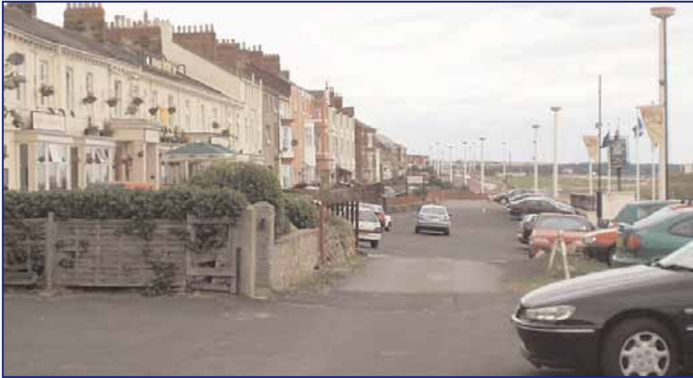
In this section of Roker Terrace almost all front gardens have been removed to accommodate car parking, detracting from the setting of these seafront properties.
