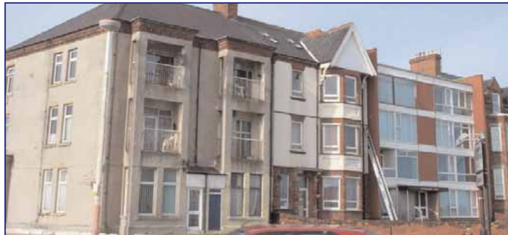
The above property, prominently located at the southern end of Roker Terrace, has been substantially altered from its original form and is in a state of disrepair. This is an unfortunate sight at the main gateway into the Conservation Area from the south and portrays a negative image of the area.
