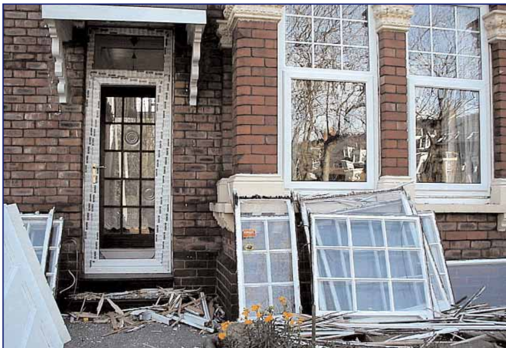
The installation of UPVC units, as illustrated above, fail to match the slender proportions and detailing of the traditional sash windows, detracting from the character of the property concerned and the terrace as a whole.
