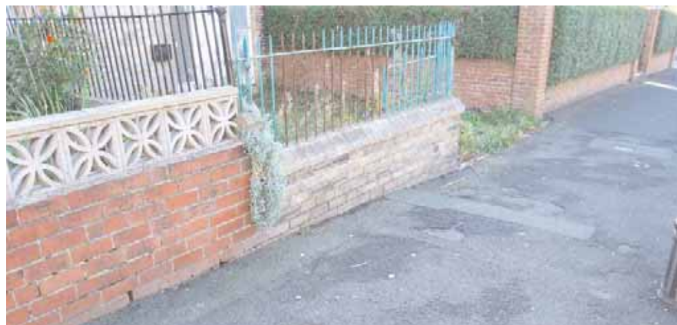
A mis-match of boundary walls and poor quality surface materials detract from the general streetscape and setting of historic buildings on the southside of Front Street.
