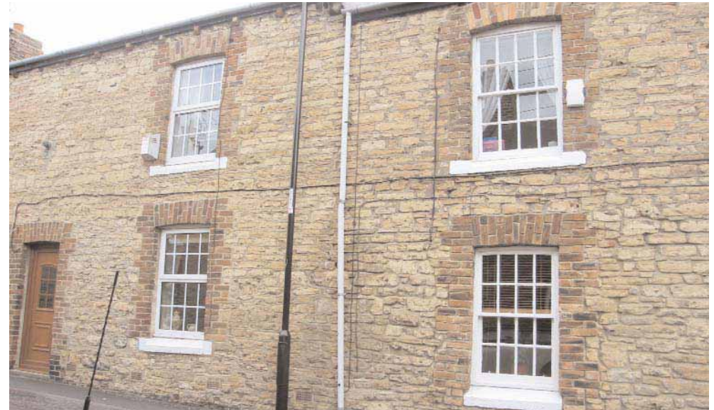
This photograph of Garden Street illustrates the difference in quality between original timber sliding-sash windows, shown to the right, and uPVC replacements to the left. The stick-on glazing bars, shiny material and thicker sections and lack of depth of the frames of the uPVC units provide a poor imitation of the original windows and detract from the historic character of the terrace.
