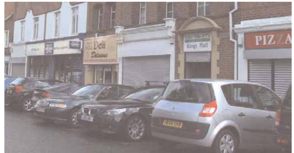
Above: modern shopfronts on Durham Road with unsympathetic signage and unattractive roller shutter security measures.
