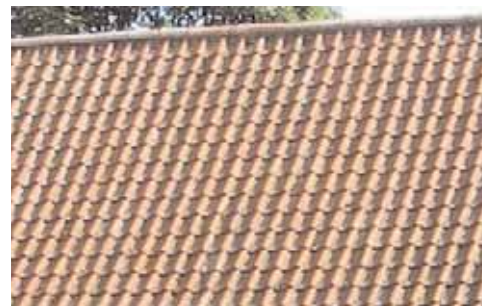
Red clay pantiles on the Almshouses
