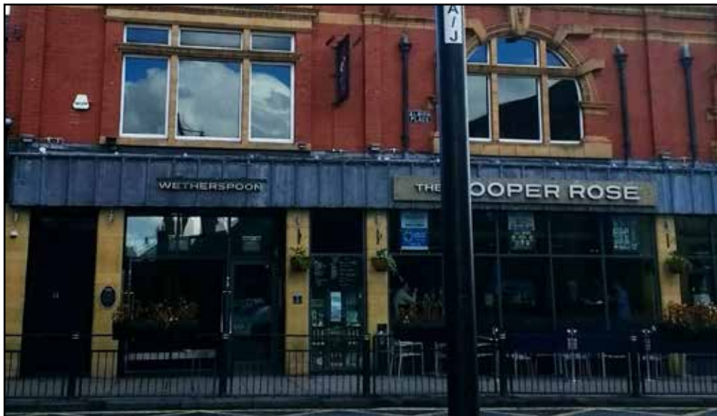
The shop front above successfully mixes traditional and contemporary materials in a simple yet high quality modern design to provide an attractive frontage that relates to the upper floor.
