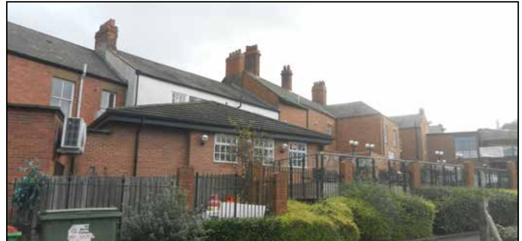
The rhythm and uniformity that originally characterised the rear of Green Terrace has been spoiled by the addition of the above extensions.
