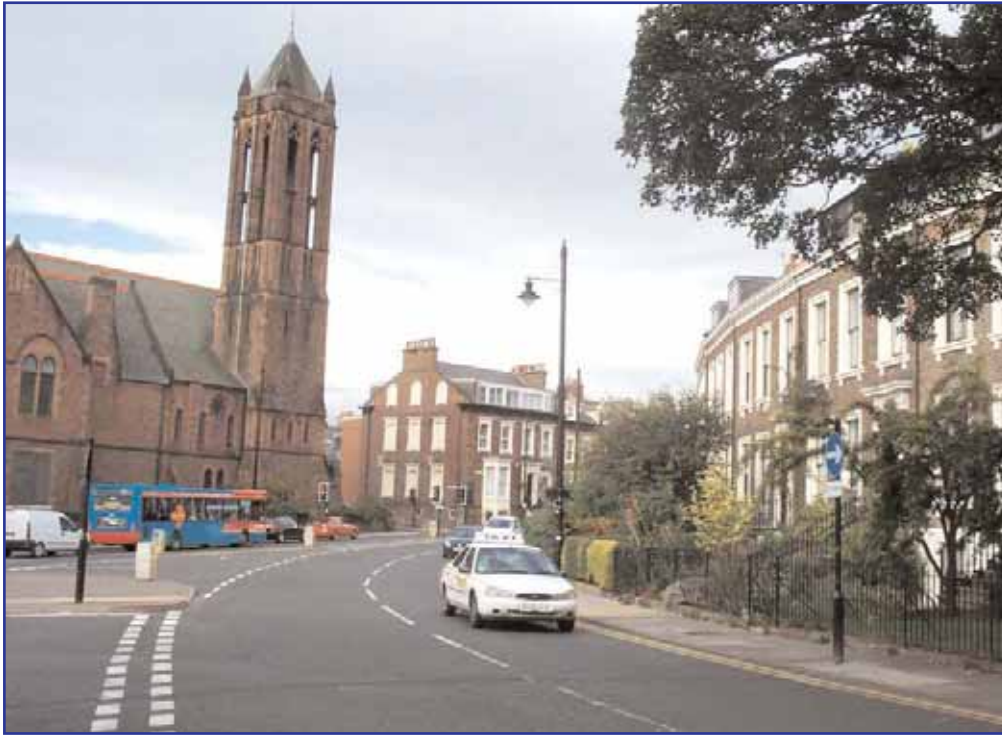
A variety of architecture, building forms and materials provides interesting contrast in the street scene, significantly enhancing its townscape value.
