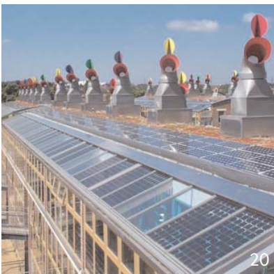
Use of photovoltaics in Bedzed, Sutton
