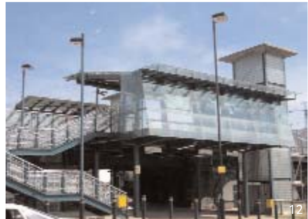
St Peter's Metro Station - Developers should consider how their scheme will link into the local public transport system.
