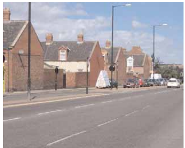
Arriving in Sunderland along Trimdon Street - a low quality environment
