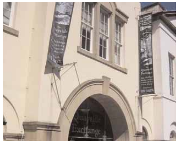
High Street West
