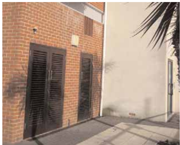
Bin storage and services are integrated into the design of this building at Gunwharf Quays in Portsmouth
