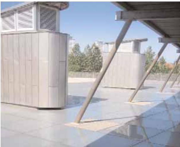
Ventilation stacks at the National Glass Centre are an integral part of the design of the building
