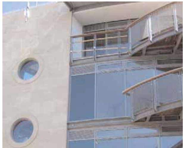
New apartments adjoining the Winter Gardens are well detailed and contemporary
