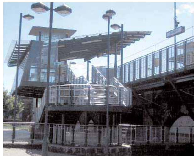
St Peter's Metro station
