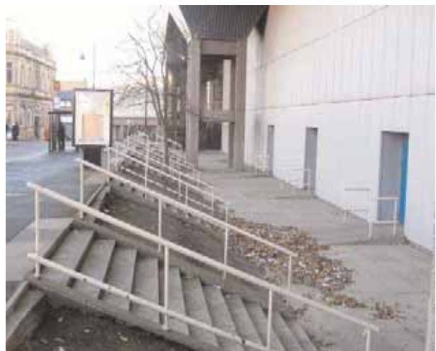
Blank elevation of Crowtree Leisure Centre
