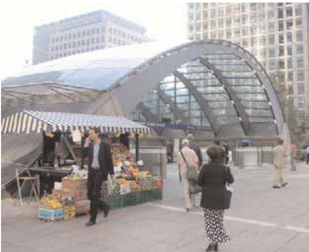
The station entrance and plaza at Canary Wharf, London make a strong, positive statement
