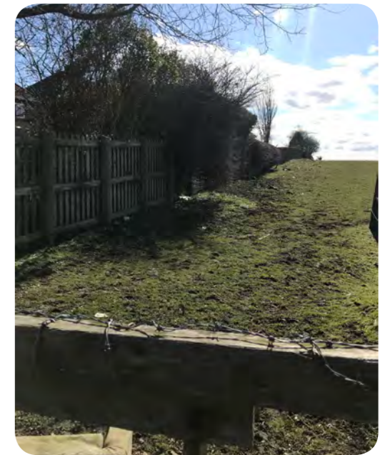
Pic.4 Back gardens of housing at Wordsworth Cres
