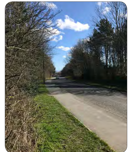
Pic.6 Stone Cellar Road main vehicular route to south
