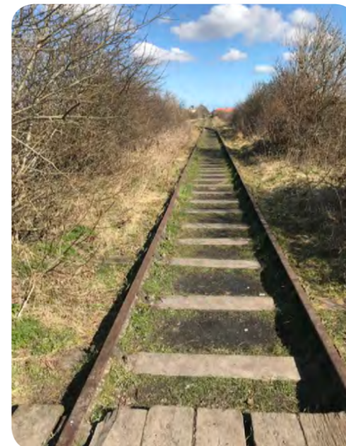
[S.A.M- Bowes Railway line]
