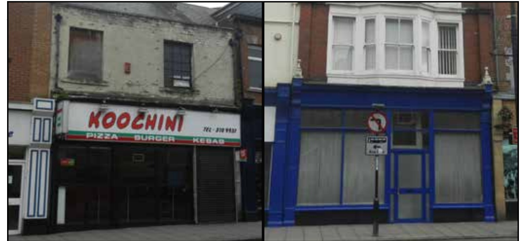
The property to the left exhibits all the defects of a poor quality, modern shop front including a plastic internally illuminated fascia, projecting box sign and external roller shutters, giving it a very poor appearance. In contrast, the premises to the right, has retained many traditional shop front features and makes a positive contribution to the historic building and street scene, though would benefit from a more traditional colour scheme.
