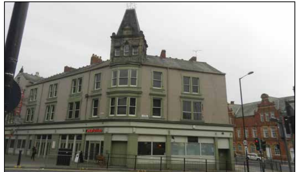
This pub frontage was formerly painted a traditional burgundy red and is now a more complimentary shade of pale green and cream
