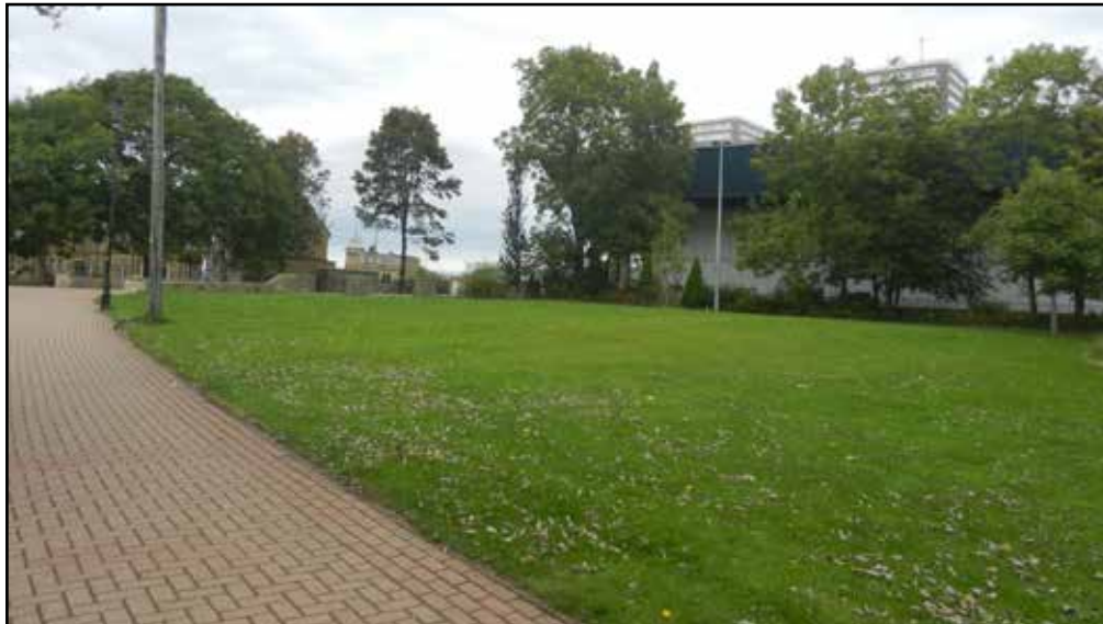
Brutal, unsightly blank elevation facing onto Town Park discourages activity and use of the space.
