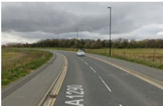
Extents of shared space unclear. Southern footway of A1290 3m wide throughout. Therefore, potential to upgrade to shared space.
