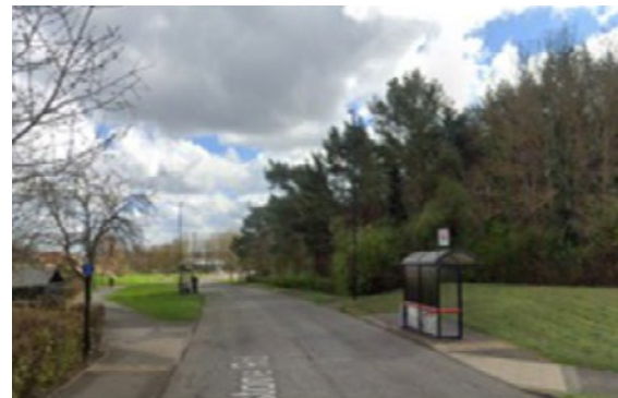
Uncontrolled shared use crossing of Silverstone Road. Multiple uncontrolled crossings on the route where traffic speeds are likely to exceed 20mph.
