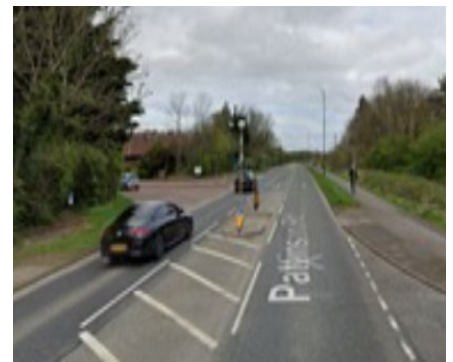
Uncontrolled crossings connections to Teal Farm and Pattinson Industrial Estate unlikely to be appropriate due to traffic speed and flow.
