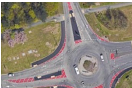
Uncontrolled crossings likely to be unsuitable at round about entry / exits.
