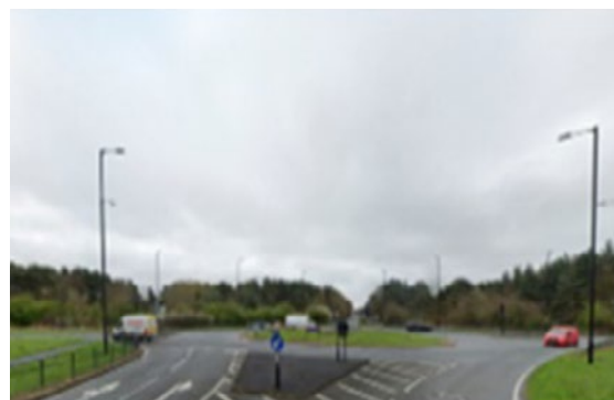
Inadequate at grade crossing facilities on the Biddick Lane roundabout. Subway alternative dark and secluded.
