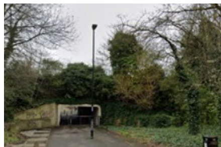
Secluded underpass with lack of lighting.
