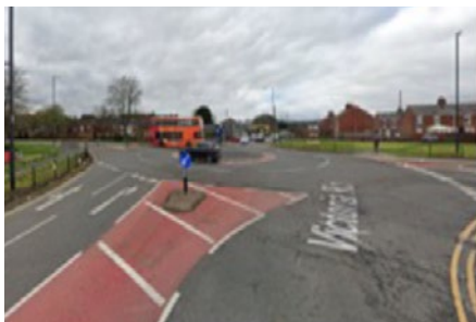
No crossings provided at key crossing location.
