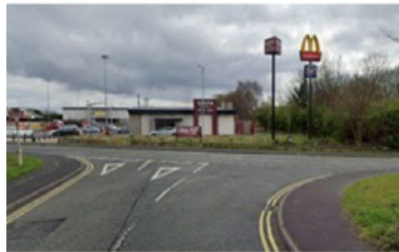
Lack of tactile paving and dropped kerbs throughout route.
