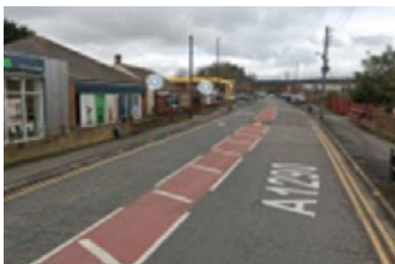
Central reserve and lack of footway likely causing higher traffic speeds.
