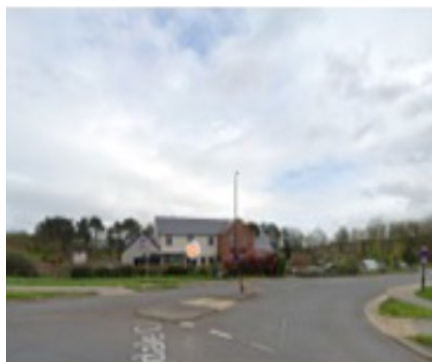
Uncontrolled crossings on roundabout unlikely to be appropriate due to traffic speed and flow.
