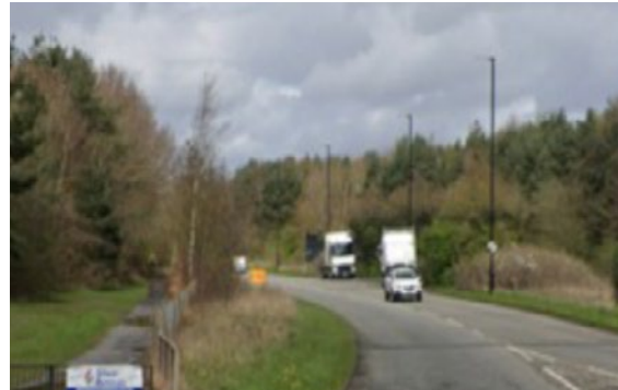
Path on west side of A195 provides shared use connectivity to Amazon de pot. However, width appears unsuitable.
