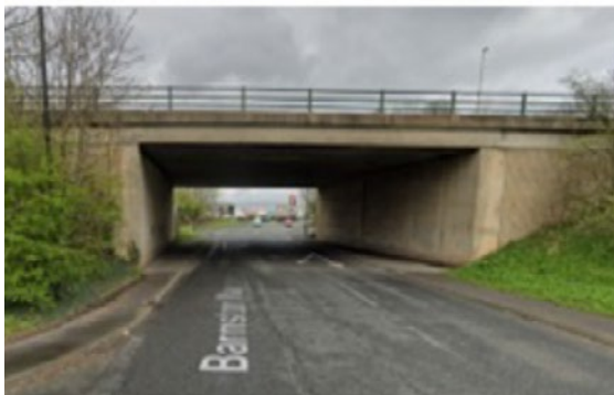
Footway widening / lighting improvements in underpass.
