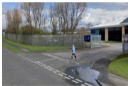
Lack of tactile paving and dropped kerbs. Signs of ponding at some crossing points.
