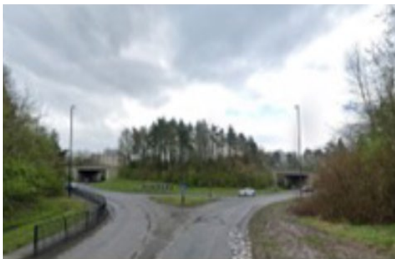
Upgrade crossing and footway facilities around Galleries South Interchange.
