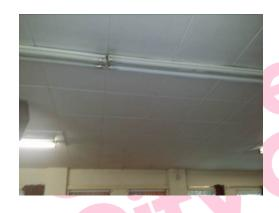
The ceiling to the hall (Room 007) contains asbestos.
