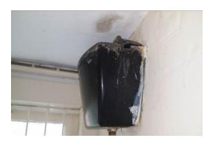
The high level cistern to the male WC (Room 005) contains asbestos.
