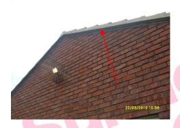
The undercloaking to the external of the building contains asbestos.
