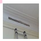
The plaster coving to ceiling/wall (Hall 1/01) does not contain asbestos.
