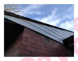
The Undercloak - to toilet block in Barnes West End Men's Pavilion – External E/001 does not contain asbestos.
