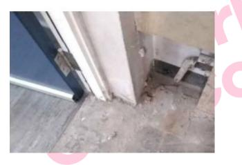
The floor tiles and adhesive in the Switch Room (Z1/001) is presumed to contain asbestos.
