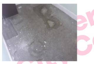
The floor adhesive under modern flooring and screed (Office Rm G/004) does not contain asbestos.
