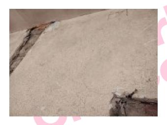
The wall coating from around the door and lintel in the outhouse (External E/006) contains asbestos.
