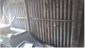
The wall sheet cladding to the garage (External E/003) does not contain asbestos.
