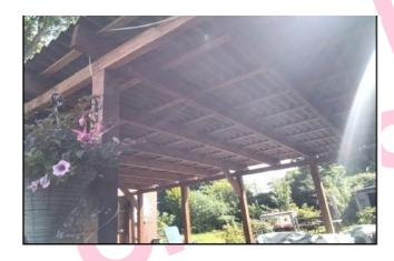
The roof – sheet cladding to the conservatory/sun room (External E/002) does not contain asbestos.
