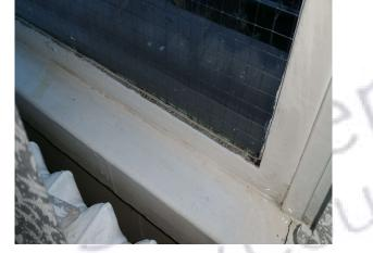
The sealant to windows in the classroom (Rm 0/13) does not contain asbestos.
