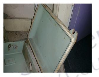
The gasket to loose lying junction box in the switchroom (Rm 1/04) does not contain asbestos.
