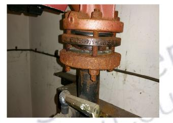
The gasket to pipework flange in the boiler room (Rm 2/10) does not contain asbestos.
