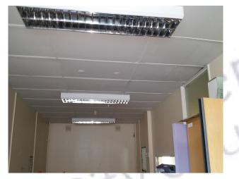
The suspended ceiling in the office (Rm 1/08) does not contain asbestos.
