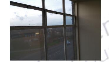
The sealant to windows in the stairwell & landing (Rm 2/01) does not contain asbestos.
