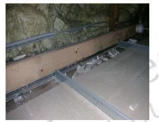
The debris to top of ceiling tiles adjacent to windows in the classroom ceiling void (Rm 0/05) does not contain asbestos.
