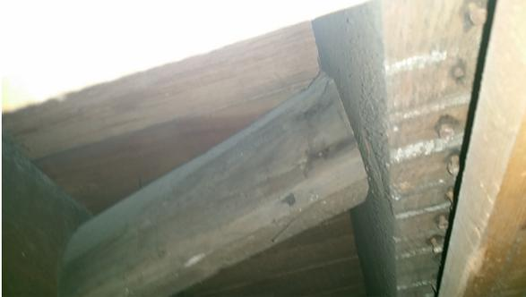
Debris to beams nails & nail holes within beams in 0/05/office (void above) do not contain asbestos.
