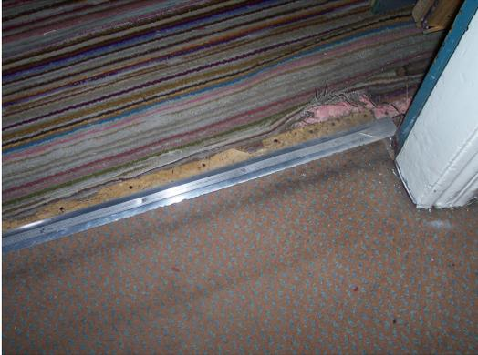
The beige flooring under carpet on corridor 3 does not contain asbestos.
