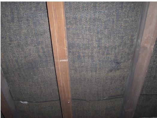
The sarking felt to roof in the loft does not contain asbestos.
