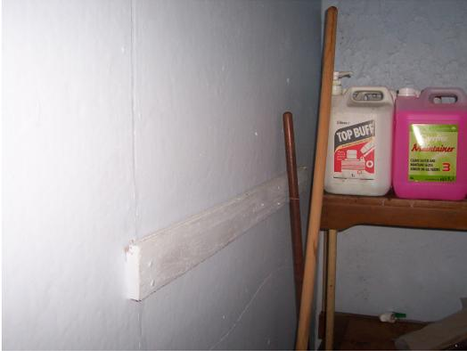
The cement panels to the walls in the cleaners store contain asbestos. Any change in its appearance should be recorded, and passed to Property Services.
