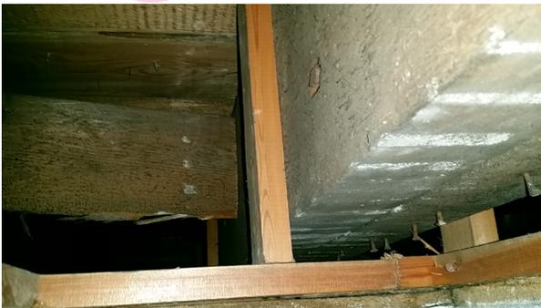
Debris to beams nails & nail holes within beams in 0/04/communal room 1 (void above) do not contain asbestos.
