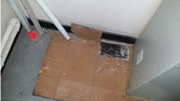
Floor tile with bitumen adhesive in 0/02/female toilets contain asbestos.
