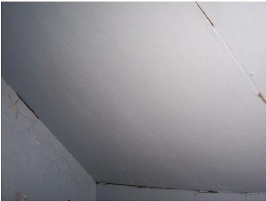
The cement panels to the ceiling angle in the cleaners store contain asbestos. Any change in its appearance should be recorded, and passed to Property Services.
