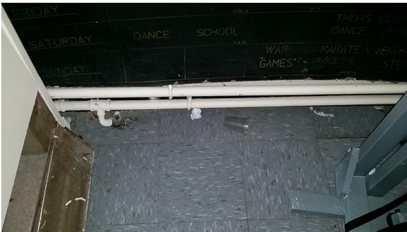
Floor tile with bitumen adhesive in 0/03/male toilets contain asbestos.
