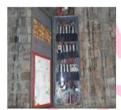
The flash guards – electrical switch gear in the Store Room (G/01) does contain asbestos.
