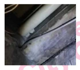
The ceiling void panel to expansion joint in the Room Lift Lobby (G/001) does not contain asbestos.
