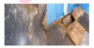
The vinyl floor to Unit 71-72 (G/01) does not contain asbestos.
