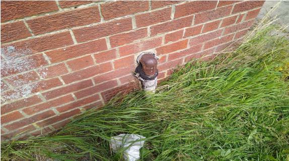
The pipe lagging (External) does not contain asbestos.
