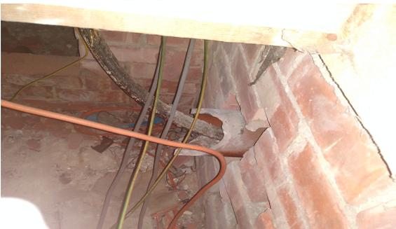
The pipe lagging floor covering in Rm 0/013 Store 2 floor void does not contain asbestos.
