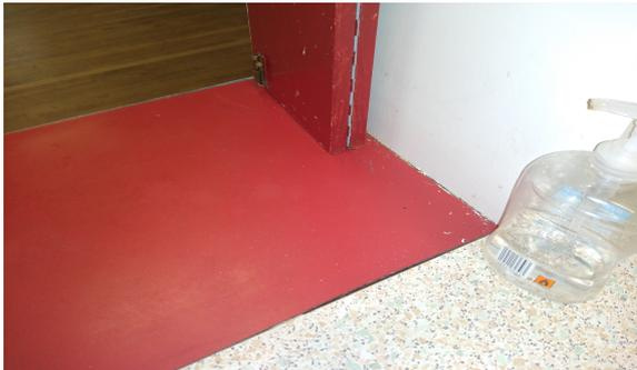
The vinyl to the serving hatch in Rm 0/012 Kitchen does not contain asbestos.
