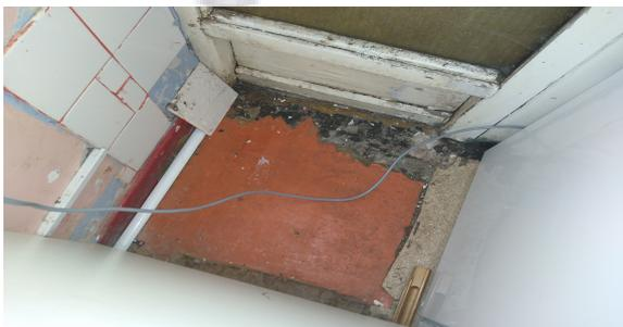
The floor covering in Rm 0/012 Kitchen contains asbestos.
