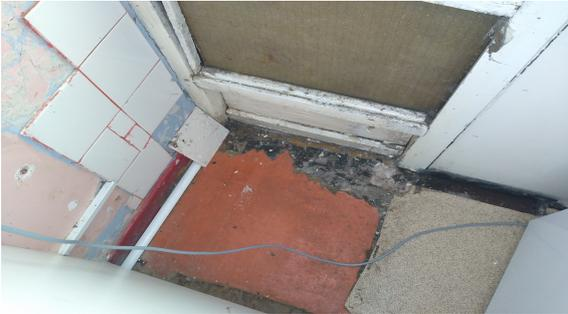
The bitumen adhesive in Rm 0/012 Kitchen contains asbestos.
