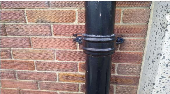
The soil pipe (External) is presumed to contain asbestos.
