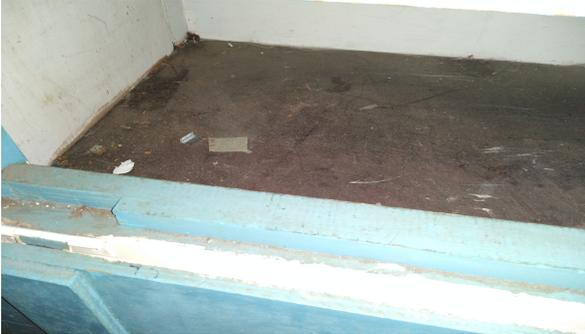
The shelf in the electric cupboard in Rm 0/004 Hall does not contain asbestos.
