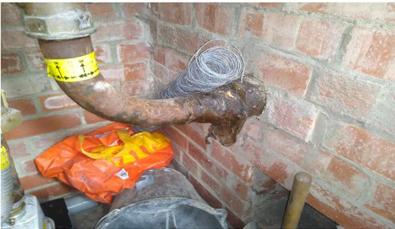
The pipe lagging in the gas store (External) does not contain asbestos.
