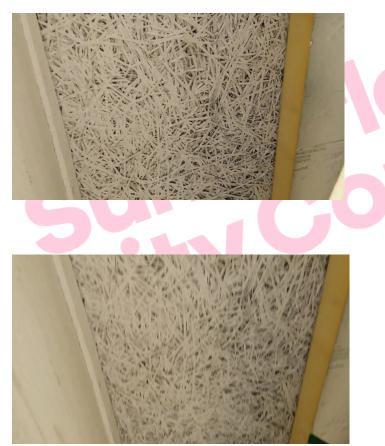
The underside of roof in Machine Wash Area -void above (Rm 0/128) does not contain asbestos.
