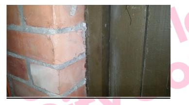
The mastic to door frame in Tank Room (Rm 1/001) contains asbestos.
