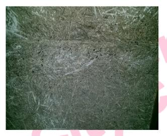
The underside of roof in Disabled Bathroom ceiling void (Rm 0/072) does not contain asbestos.
