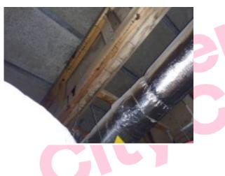
The bitumen drip walls and roof structure in Office 38a (G/033) does not contain asbestos.
