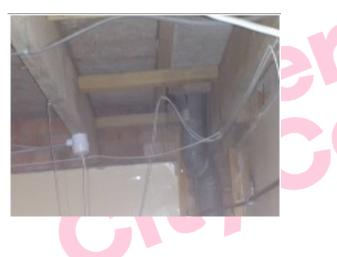
The bitumen drip walls and roof structure in the Female Toilets (G/058) does not contain asbestos.
