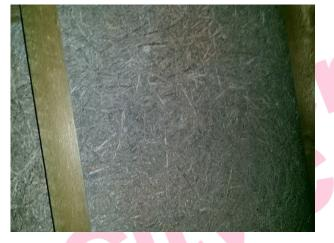
The underside of roof in Duty Office ceiling void (Rm 0/073) does not contain asbestos.
