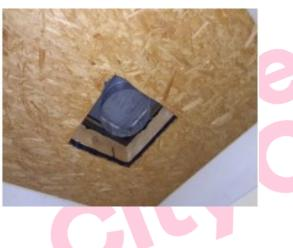
The bitumen drip skylight roof cover in the Drop-in room B (G/06) does not contain asbestos.
