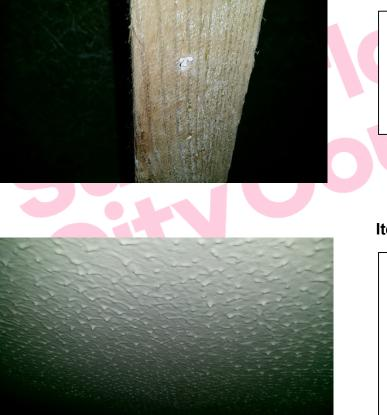
The debris to beams in Disabled Toilet-void above (Rm 0/104) does not contain asbestos.
