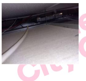
The textured coating debris – top of ceiling tiles and light fittings in Meeting Room 1 (G/02) does contain asbestos.
