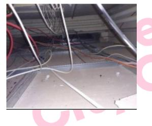
The textured coating debris – top of ceiling tiles and light fittings in the Corridor (G/049) does not contain asbestos.
