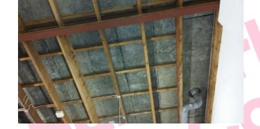
The underside of roof in Equipment Store (Rm 0/135) does not contain asbestos.
