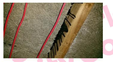
The underside of roof in Corridor-void above (Rm 0/098) does not contain asbestos.
