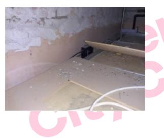
The textured coating debris – top of ceiling tiles and light fittings in Store cupboard 32 (G/038) does not contain asbestos.
