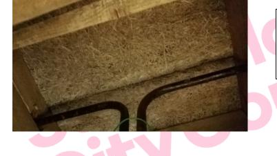
The underside of roof in Male Toilet -void above (Rm 0/108) does not contain asbestos.
