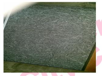
The underside of roof in Male Toilets & Lobby ceiling void (Rm 0/071) does not contain asbestos.
