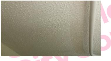
The textured coating to ceiling in Photocopier Rm-void above (Rm 0/102) contains asbestos.
