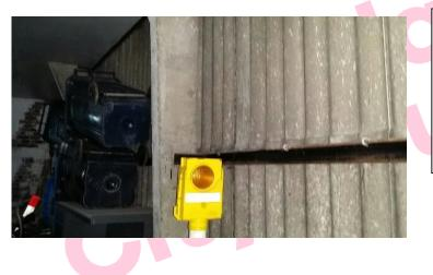
The wall cladding in the Salt Shed (Rm 0/44) contains asbestos.
