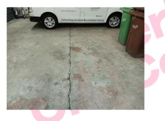
The putty on floor in Area 4/Garage and Store Area does not contain asbestos.
