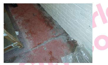
The putty to joints in floor in Area 1/Store Room does not contain asbestos.
