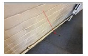
The tile debris under modern tile in the Mess Room (G/01) does not contain asbestos.
