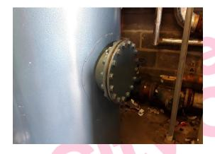
The vessels tank gasket (Area 36/Boiler Room) does not contain asbestos.
