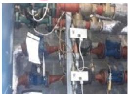
The pipework gasket to pipework V12 right side (Boiler Room G/001 – The Oval) does contain asbestos.
