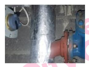
The pipework gasket to pipework V12 left side (Boiler Room G/001 – The Oval) does contain asbestos.
