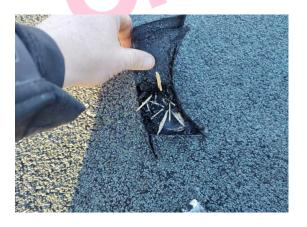
The floor - felt roof (Bitumen) (Area: 1 Roof 1) does not contain asbestos.
