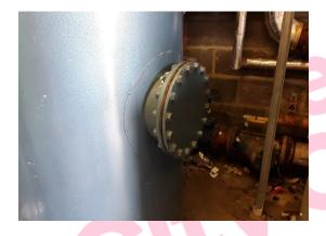
The vessels tank gasket (Area 36/Boiler Room) does not contain asbestos.
