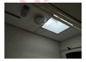
The ceiling (Textile) (Area: 9 Disabled WC) contains asbestos.
