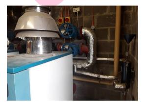
The pipe flanges (Area 36/Boiler Room) contain asbestos.
