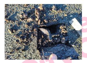
The floor - felt roof (Bitumen) (Area: 2 Roof 2) does not contain asbestos.
