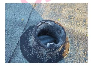
The flue (Area: 1 Roof 1) contains asbestos.
