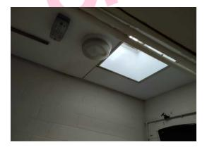
The ceiling (Textile) (Area: 9 Disabled WC) contains asbestos.
