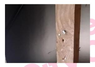
The minor sporadic residue to existing nails in the ceiling (Area 2/Annexe room ceiling void) does contain asbestos.
