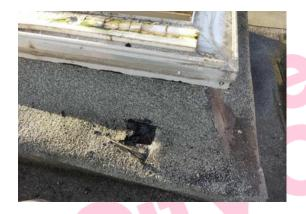
The bitumen felt roof lining (external/Roof 1) does not contain asbestos.
