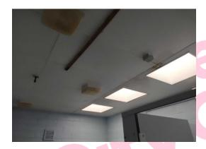
The ceiling (Textile) (Area: 8 Male WC) contains asbestos.
