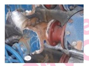
The pipework gasket to pipework V6 right side (Boiler Room G/001 – The Oval) does contain asbestos.
