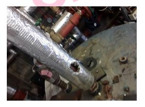
The redundant gaskets on top of tank (Area 36/Boiler Room) do not contain asbestos.
