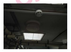
The ceiling - paper lined fibreboard ceiling tiles (Textile) (Area: 6 Caretakers Cupboard) contains asbestos.
