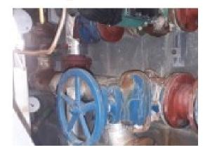
The pipework gasket to pipework V8 left side (Boiler Room G/001 – The Oval) does contain asbestos.
