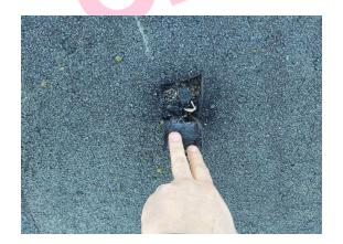
The floor - felt roof (Bitumen) (Area: 1 Roof 1) does not contain asbestos.
