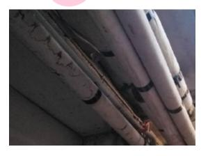
The pipework insulation in the store cupboards (Room 014/A) does not contain asbestos.
