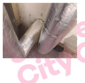
The debris/residue to floor and unlagged pipes Ground Floor, Cupboard, G.001 contains asbestos.
