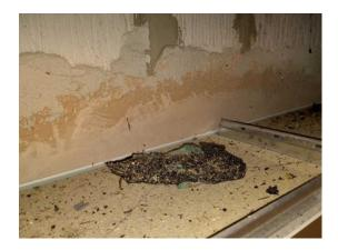
The ceiling (Area 29/Toilet) does not contain asbestos.
