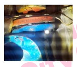
The Gaskets pipework RHS side (Keystage 1 Plant Room G/01) does not contain asbestos.
