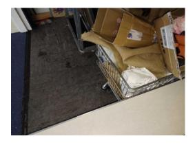
The floor (Area 82a/Store Cupboards) contains asbestos.
