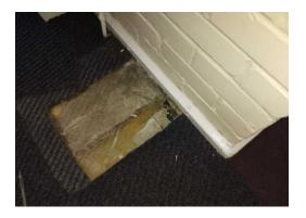
The floor (Area 72/Corridor) does not contain asbestos.
