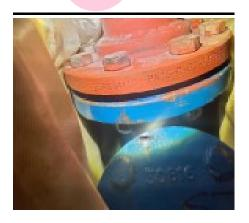
The - Gaskets pipework at high level and behind plant RHS side (Keystage 1 Plant Room G/01) does not contain asbestos.
