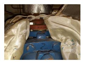
The gaskets (Area 105/Tank Room) do not contain asbestos.
