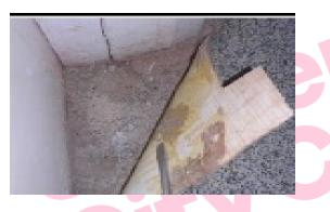
The residual adhesive beneath modern vinyl and screed in the reception lobby (G/01) does not contain asbestos.
