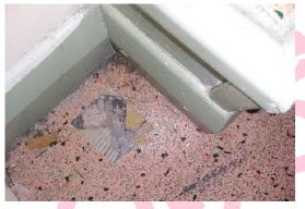
The residual adhesive beneath modern vinyl and screed (Early Years WC 2 /Area 2) does contain asbestos.
