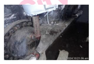
The residual insulation to copper tank front flanges x 2 (Boiler Room/Area 001) does contain asbestos.
