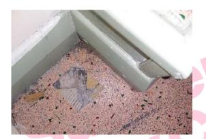
The residual adhesive beneath modern vinyl and screed (Reception Class /Area 5) does contain asbestos.
